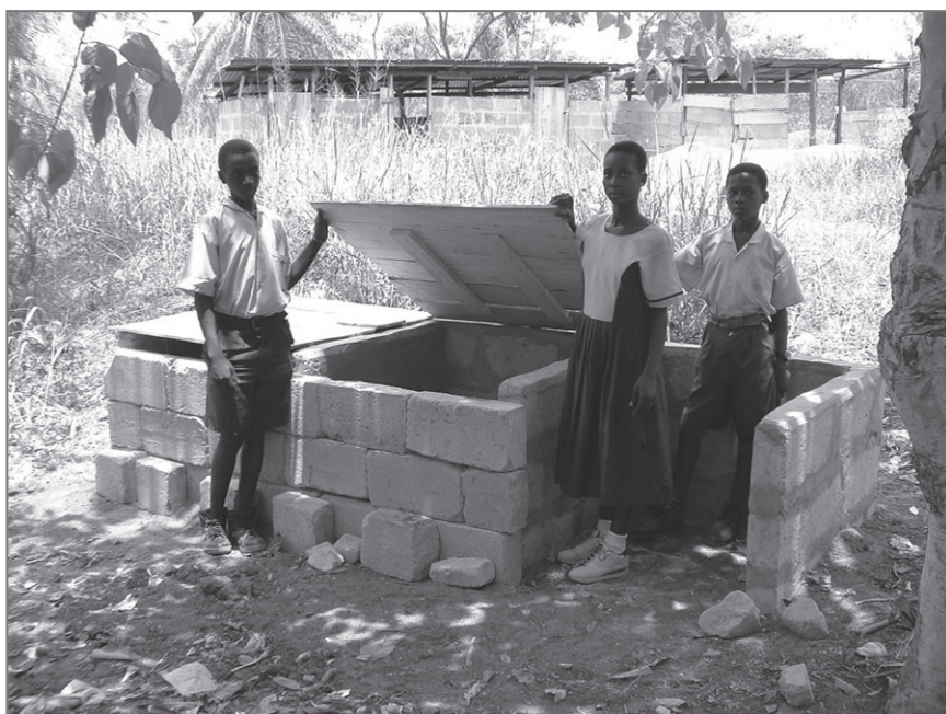
Figure 2. Double chamber (top) and triple chamber (bottom) block-built compost containers.
