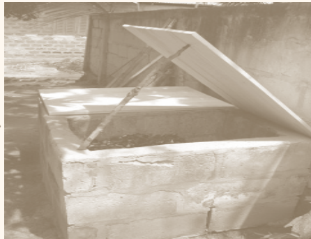
Block-built double chamber compost bin in Esereso, Kumasi
