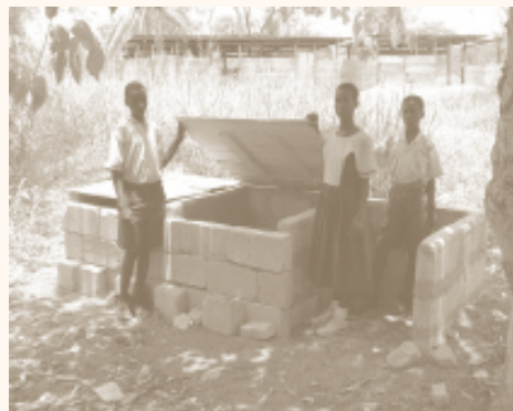
Block-built triple chamber compost bin being used at Apeadu Junior Secondary School, Kumasi
